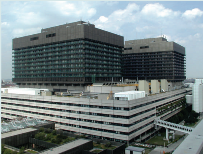
AKH Vienna (source: AKH information centre)
