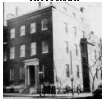
Campus of the Columbia College of Chiropractic in Baltimore (Miscellany, 1985)
