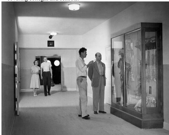
Portion of the main entrance hall – Some eighty feet long, this corridor, which was specially designed by Walter J. Kelly, prominent architect, permits rapid transit between the various departments and class rooms.
