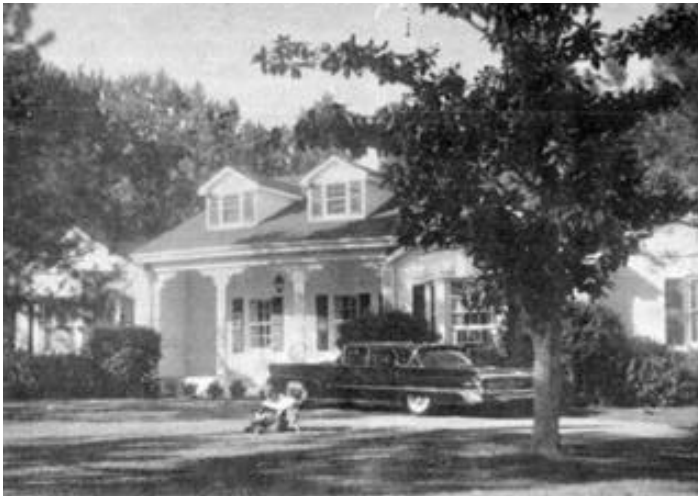
“Front view of the Harris Residence located on the outskirts at Albany on a half acre of land”
